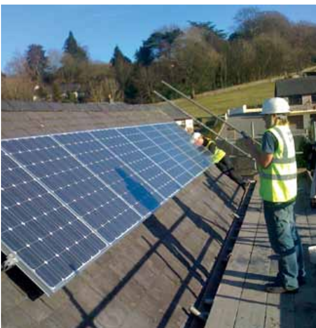
Integrated solar PV on a new build in south Scotland (Photo: Sundog Energy Ltd.)
