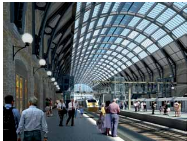
PV glazing project on King’s Cross station (impression) (Photo: Sundog Energy Ltd)
